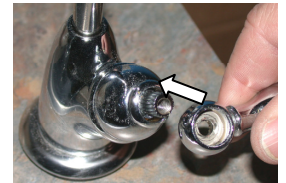
8. Hand-tighten cartridge cap and place handle back to position. Note: Check handle position to verify that the handle is fully vertical in the ON position and horizontal in the OFF position. Remove and re-position if necessary
