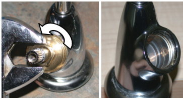
6. Using a wrench unscrew the cartridge from the faucet body & discard old cartridge
