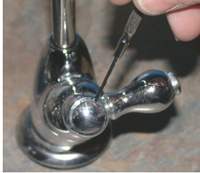
3. Pry open the handle hole cover with a small flat-head screwdriver or a similar tool.
