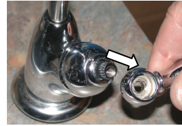
5. Pull the handle off the body and unscrew the cartridge cap by hand.
