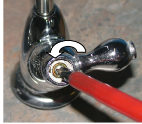
4. Unscrew the handle screw with a Philips # 2 screwdriver
