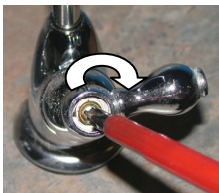
9. Screw on the handle screw & tighten.
