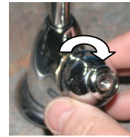
8. Hand-tighten cartridge cap and place handle back to position. Note: Check handle position to verify that the handle is fully vertical in the ON position and horizontal in the OFF position. Remove and re-position if necessary
