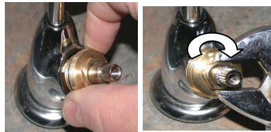
7. Screw on the new cartridge into the faucet body and slightly tighten it using a wrench. Caution: Do not over tighten
